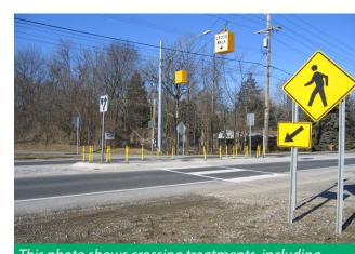
This photo shows crossing treatments, including overhead and roadside signage, pavement markings, and a refuge island for a segment of the Clinton River Trail in Oakland County.
